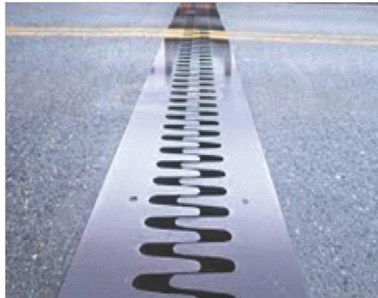
Fig.10.5: (a) Expansion gaps in railway tracks (b) Expansion joints in bridges
